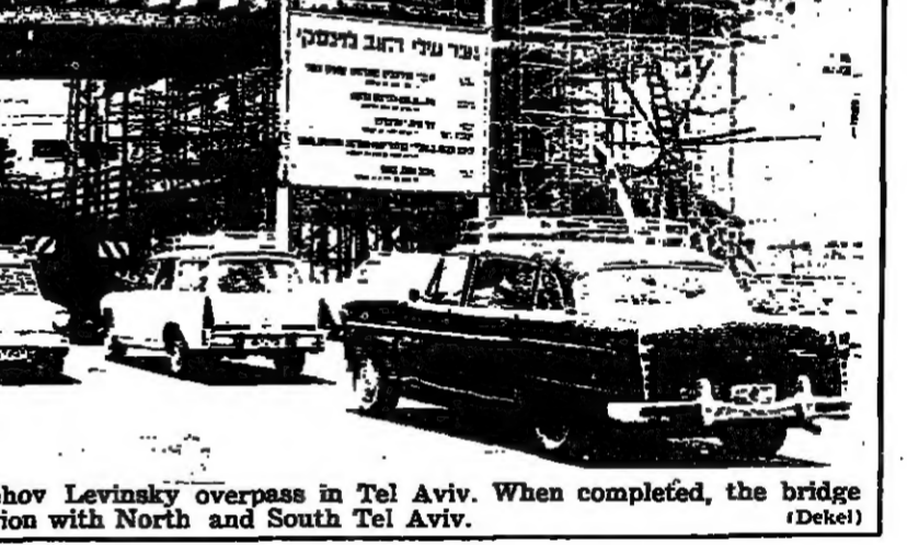
Construction has begun on the Rehov Levinsky overpass in Tel Aviv. When completed, the bridge will connect the new central bus station with North and South Tel Aviv. (Dekel)
